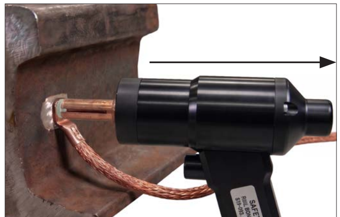
6. After finished brazing, wait 3 seconds and pull the gun straight back without pulling the trigger.
