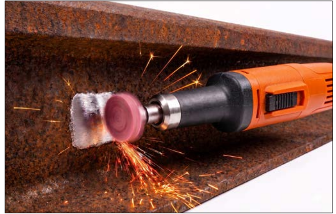
2. Grind the brazing area.
