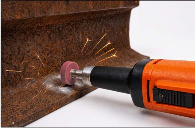
1. Grind the grounding area.
