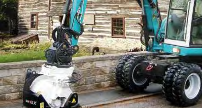
PLB 450. Footpath milling.
